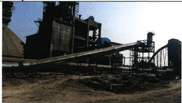
Gypsum Belt Conveyor to Cement mill
