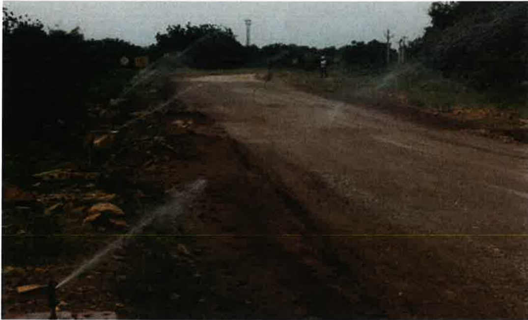
WATER SPRINKLERS IN MINES HAULAGE ROAD
